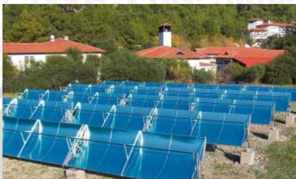
Gambar 2.1 Pemanas air tenaga surya tipe cylindrical parabolic collector Sumber: Process Heat Collector , (Weis & Rommel, 2008:18)
