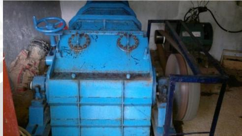
Gambar 2.11. Turbin *Cross Flow* C4-20
