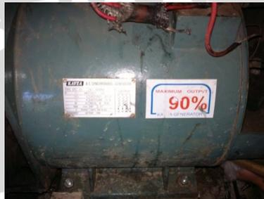
Gambar 2.8. Generator Sinkron
