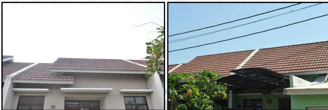
Gambar 4.12 Kualitas Atap Rumah di Perumahan Kahuripan Nirwana Village
