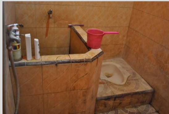
Gambar 4.52 Perubahan Toilet di Perumahan Kahuripan Nirwana Village
