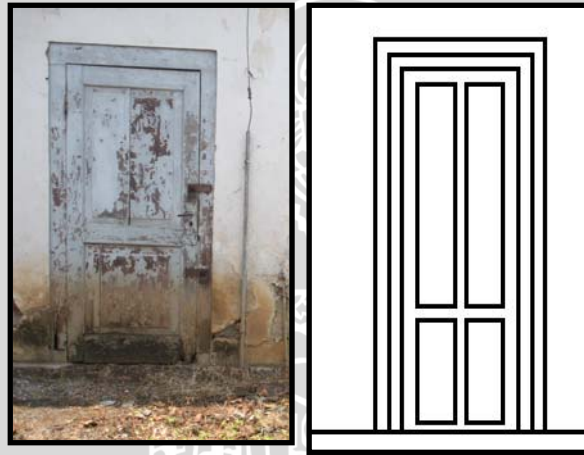
Gambar 4.130. Pintu bangunan engineering
