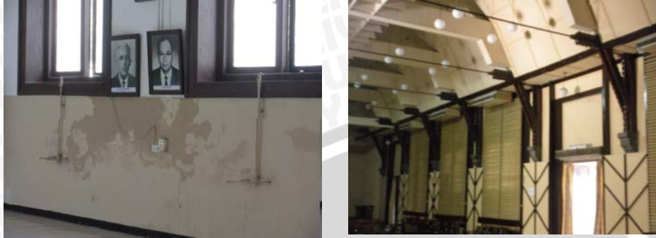
Gambar 4.15. Dinding interior museum
