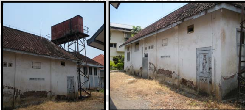
Gambar 4.129. Dinding bangunan engineering
