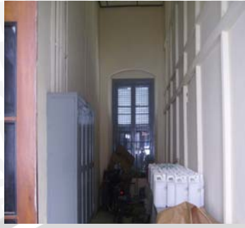
Gambar 4.149. Dinding laboratorium bibit
