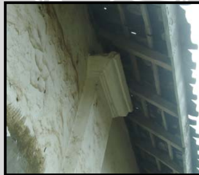
Gambar 4.132. Ornamen bangunan engineering
