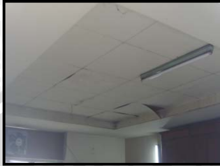
Gambar 4.145. Plafond interior Pengadaan
