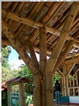
**Gambar 53.** Cam connection
