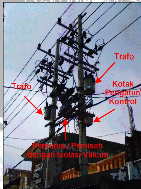
Gambar 2.14 Automatic Vacuum Switch (AVS)
