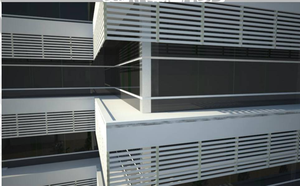
**Gambar 4. 65 sun shading**
