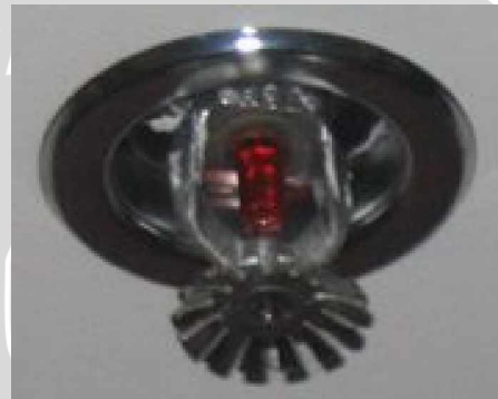
Gambar 2.3 Sprinkler Head
