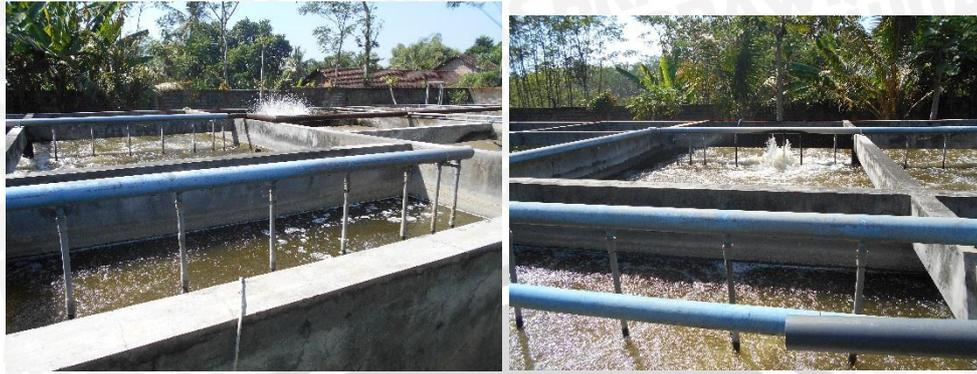
**Gambar 68.** Reaktor aerob
