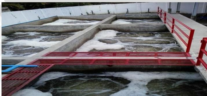
**Gambar 10.** Bak Reaktor Aerob
