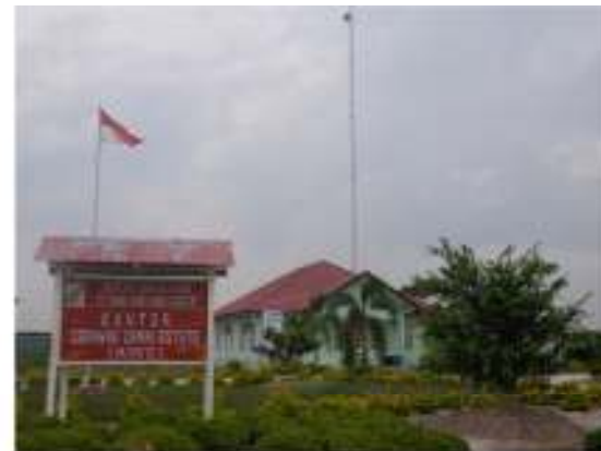
Gambar 11. Kantor Serawak Damai Estate (foto: Aditama, 2012)
