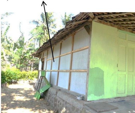
Gambar 4.24 Dinding triplek
