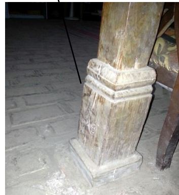
Gambar 4.48 Pondasi umpak
