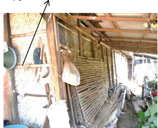
Gambar 4.25 Dinding bambu
