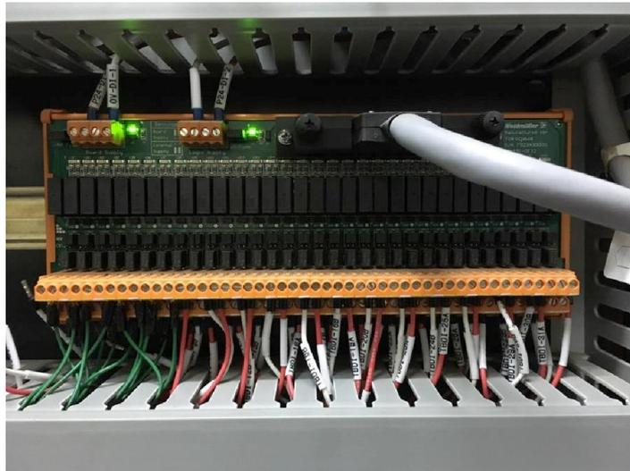
Gambar 3.5 Port Output Digital DCS
