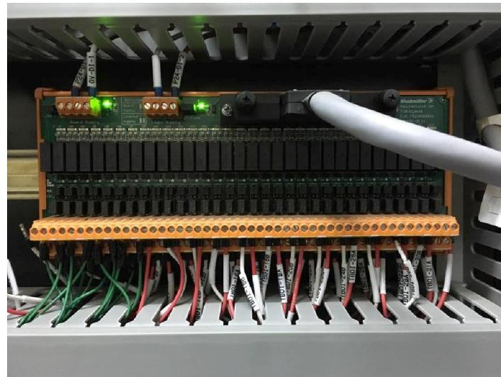
Gambar 3.5 Port Output Digital DCS
