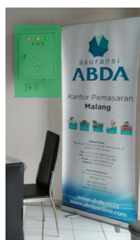
Gambar. 4.256 Box MCB Lantai 1
