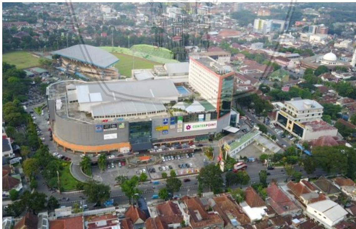
Gambar 4.1 Mall Olympic Garden
