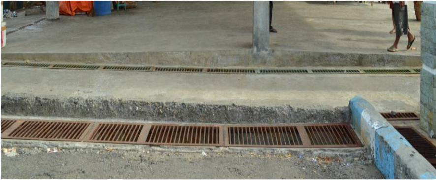
Picture 10: Water Channel Source :PPI Popoh
