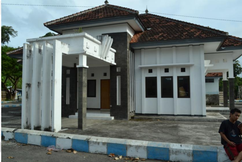
Picture 18: PPI Popoh Multifunction Building Source: PPI Popoh, 2013
