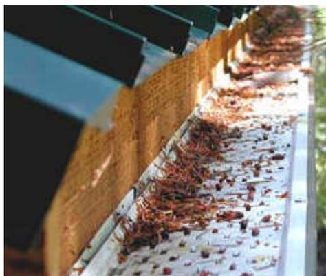
*Gambar 2. 8* Gutter guard
