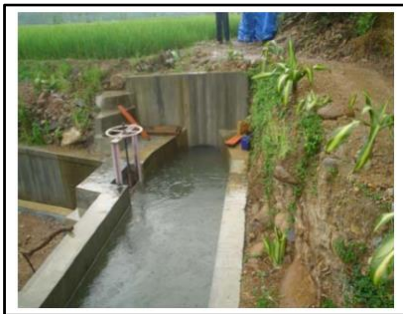
Gambar 2.39 Bak Pengendap ( Settling Basi ) Sumber: JICA (2009:2-2)
