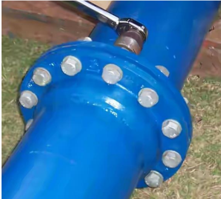
Gambar 2.6. Flange Joint
