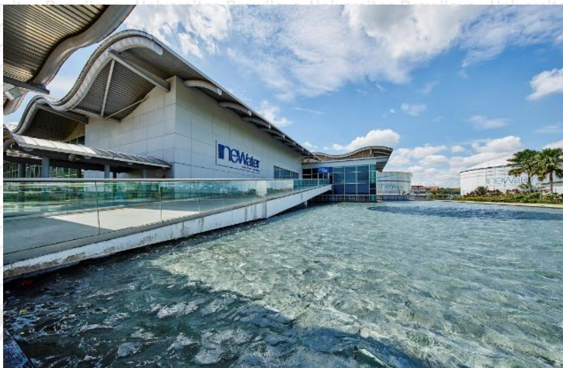
Gambar 5.8 NEWater Visitor Centre (sumber: https://www.pub.gov.sg/watersupply/fournationaltaps/newater )
