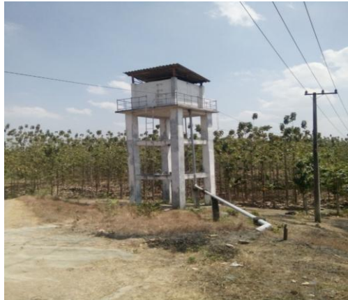
Gambar 4.18 Tandon Air Permanen Swadaya
