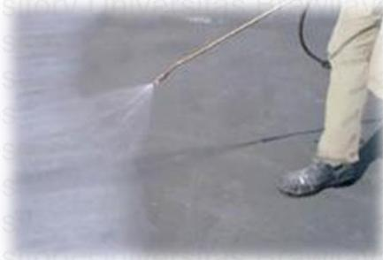
Gambar 4.80 *Precooling of Concrete*
