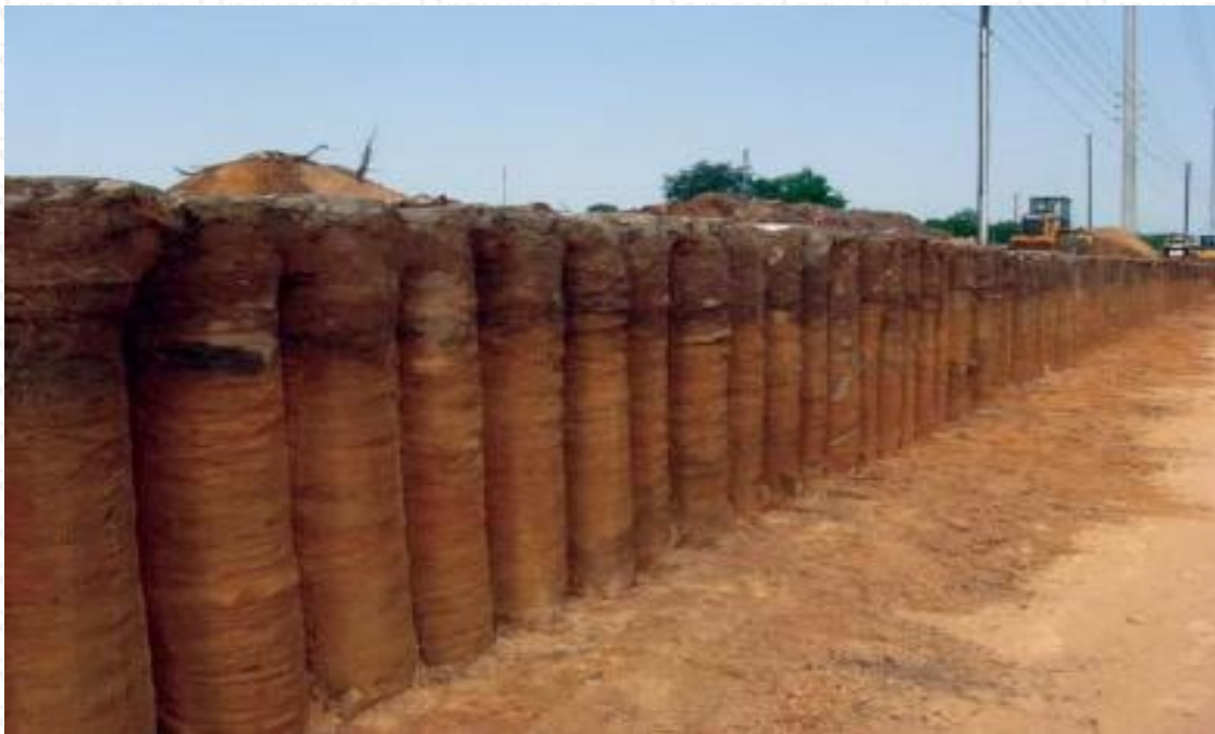
Gambar 2.5 Kolom stabilisasi hasil deep soil mixing
