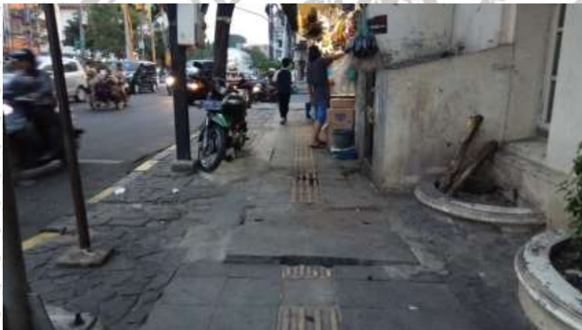
Gambar. 4.44 Kondisi Guiding blocks segmen 4
