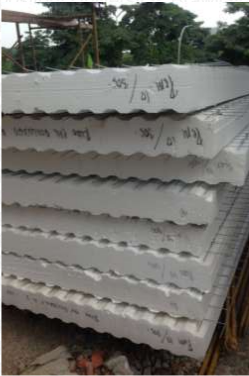
Gambar 1. Single Panel Tipe PSM 10
