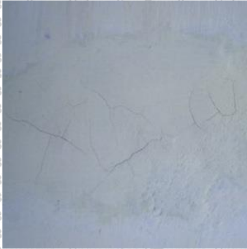
Gambar 2. 17 Map Cracking
