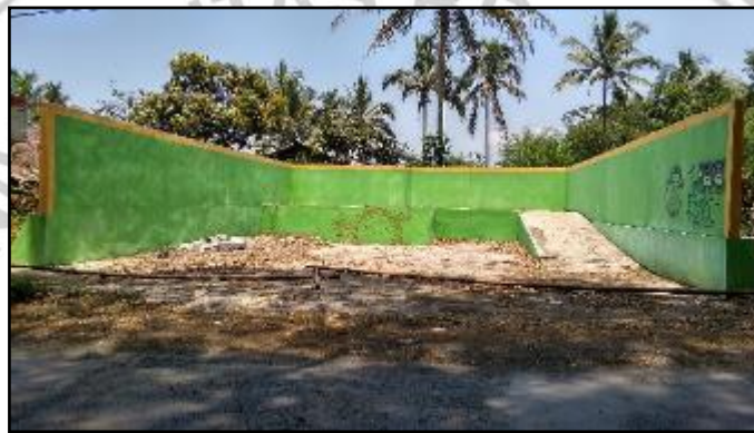
Gambar 4. 24 Kondisi TPS Cemorokandang Sumber: Survei Primer, 2019
