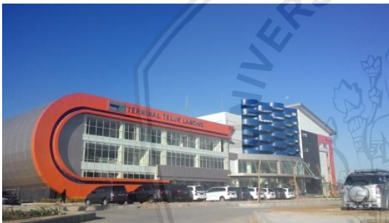
Gambar 4.8 Main building PT Terminal Teluk Lamong
