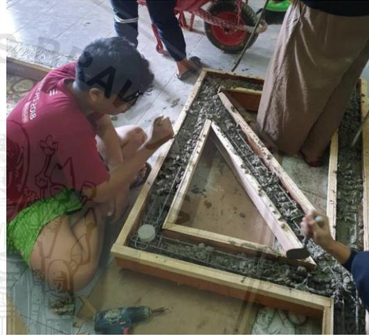
Gambar L 4.11 Proses pengecoran bekisting
