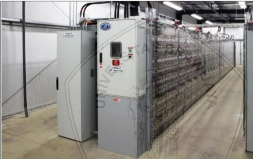
Gambar 1.1 Sistem *Redox Flow Battery* di stasiun kota Lyon (May dkk., 2018)
