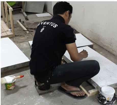
Gambar L 4.17 Proses pengecatan panel beton
