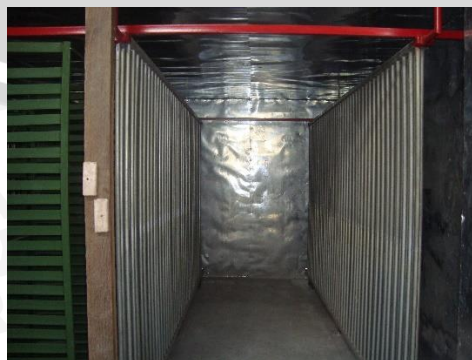
Gambar 4.2 Fire Tube Boiler dan Room Dryer Sumber: CV XYZ
