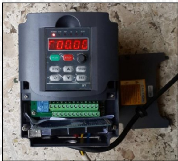
Variable Frequency Drive (VFD)
