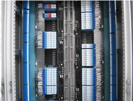
Gambar 2.7 I/O Module DCS (Sumber: https://thecontrolblog.com )
