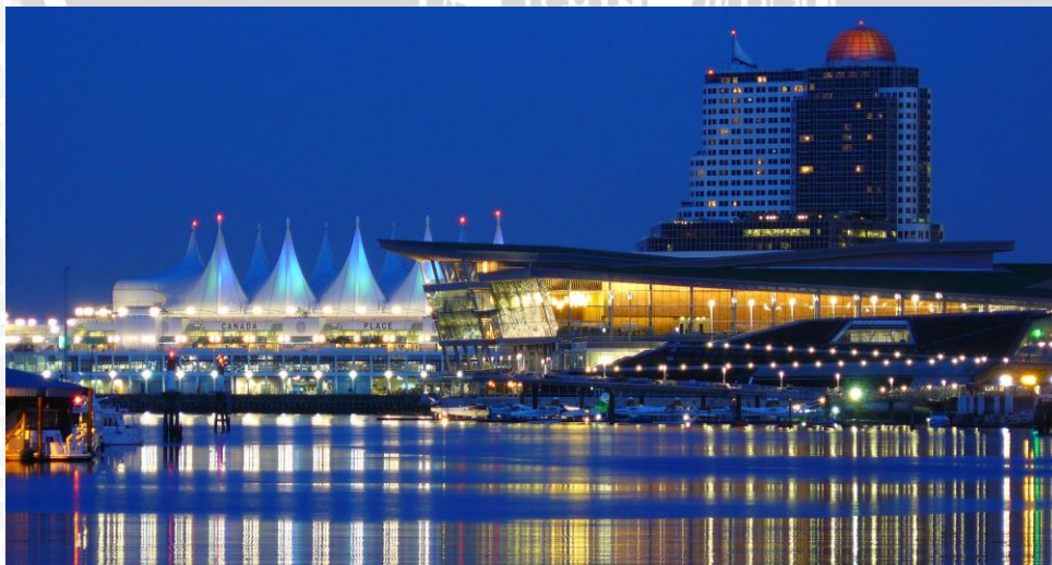
Gambar 2. 1 Vancouver Convention Center East & West Building (Sumber: www.google.com )
