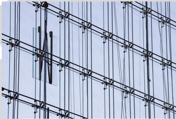
Gambar 2.8 Curtain Wall System
