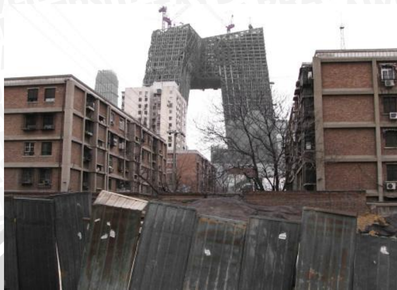
Gambar 2.23 CCTV under construction in 2008
