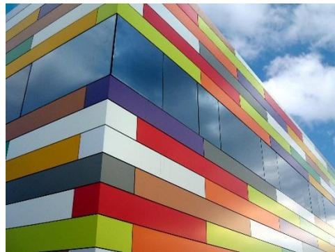
**Gambar 2.50. Aluminium composite panel**
