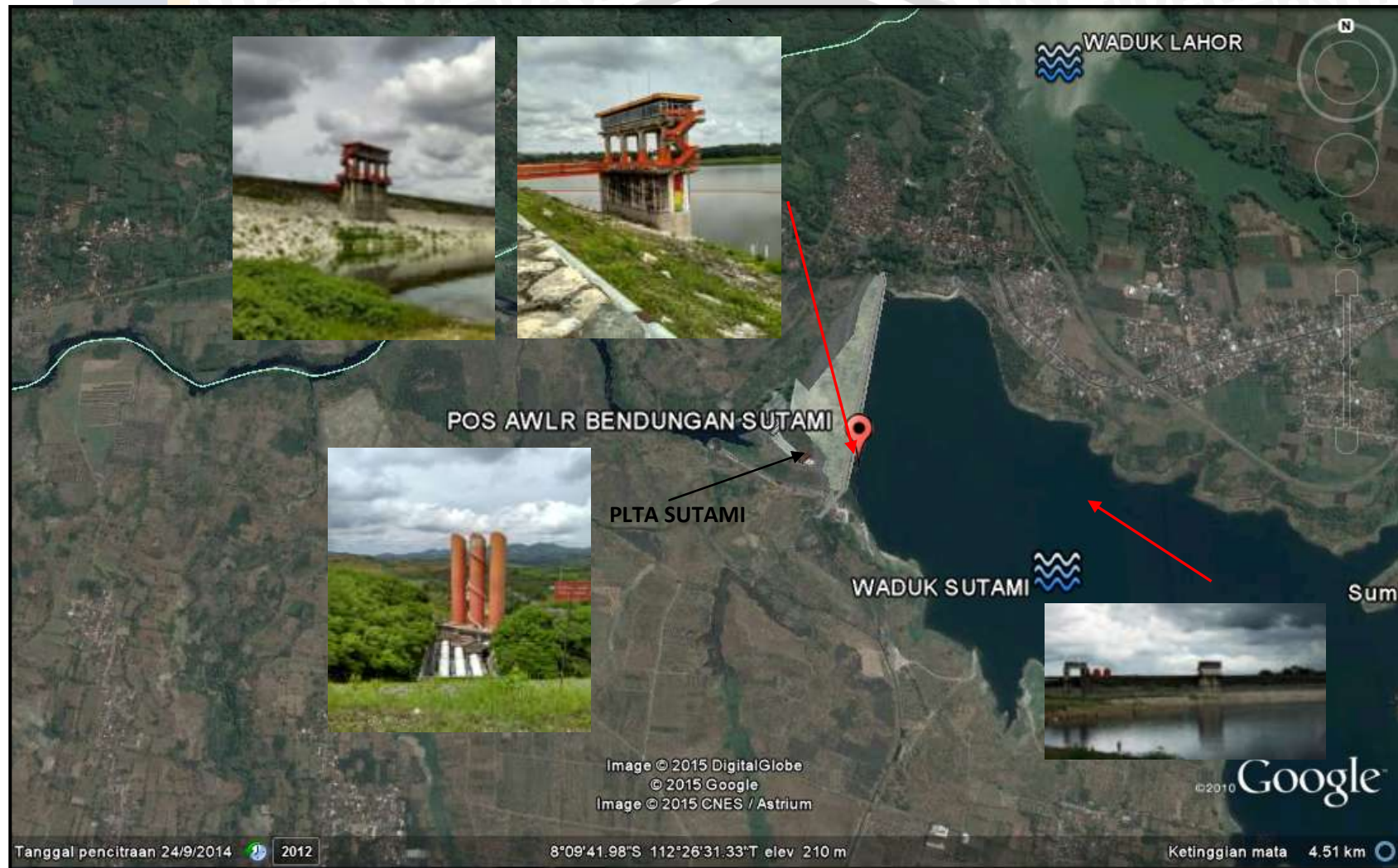
Gambar 3.2. Pos AWLR (Automatic Water Level Recorder) Waduk Sutami (Sumber: Dokumentasi 2015)
