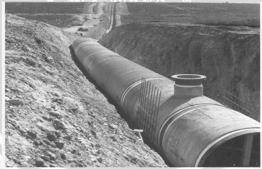
Gambar 2.15. Pipa pesat tertanam (Sumber : Bambei, 1996: 4)
