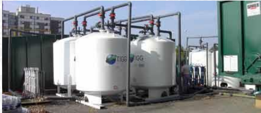
Gambar 4.38 Ground Water Treatment
