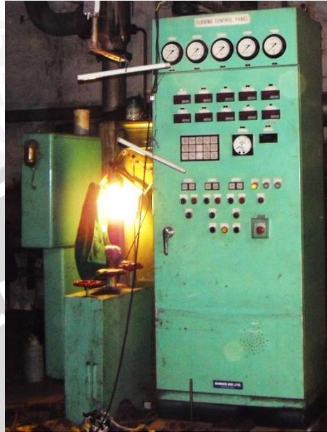
**Gambar 4.7** Turbine Control Panel Shinko
