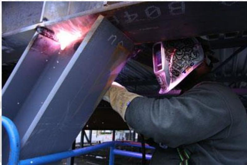
Gambar 4.23 *Overhead Welding*
