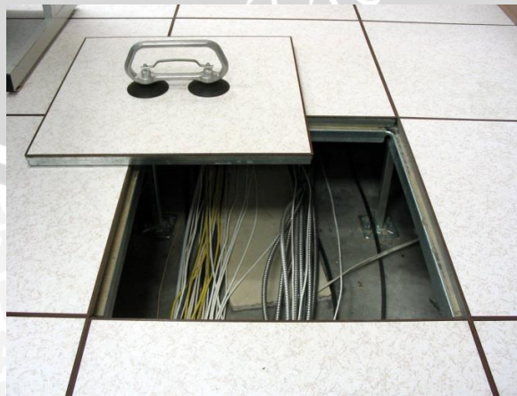
Gambar 2.5. Lantai access floor (Sumber : Gatut Susanta, 2008)
