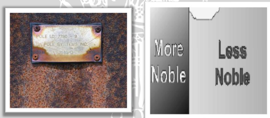
Gambar 2.14 Korosi galvanik ( galvanic corrosion )
