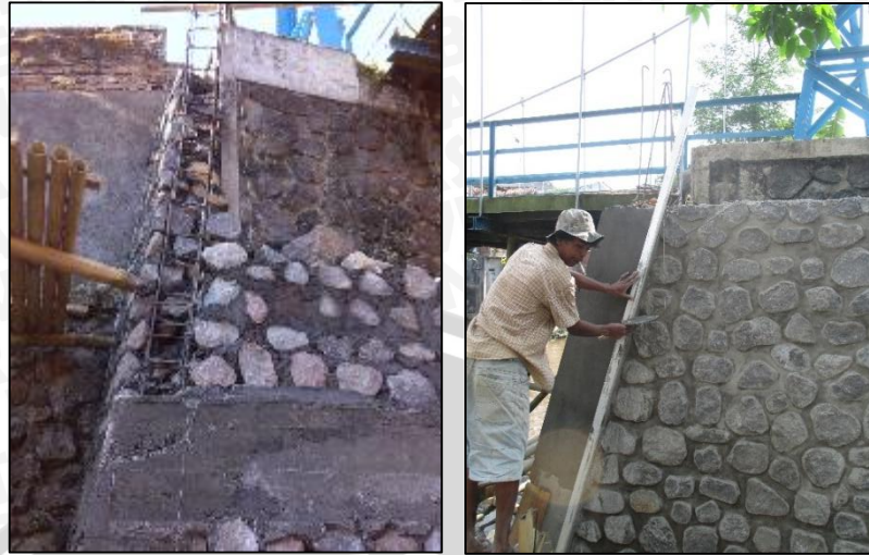
Gambar 4.34 Proses pekerjaan abutment
