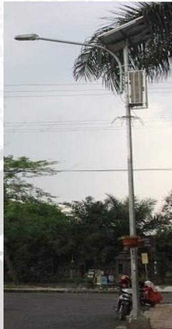
Gambar 2.22 Tiang Lampu PJU jenis Octagonal LED Sumber : Hasil Survey PJU
