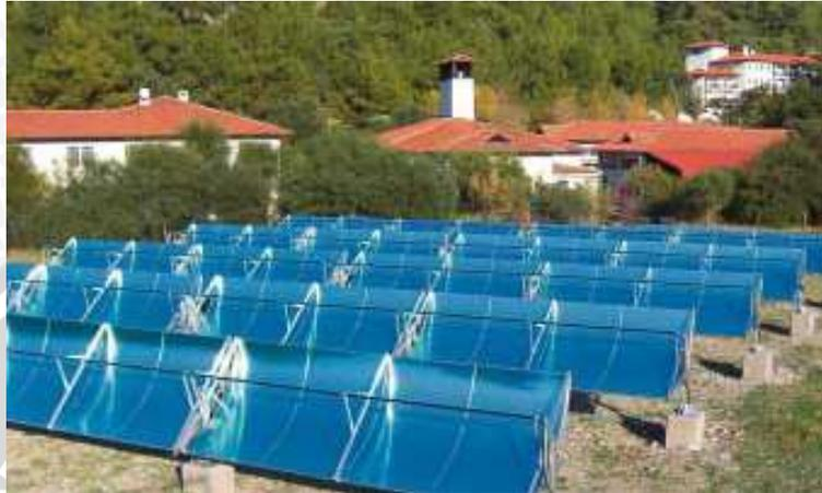
Gambar 2.1 Pemanas air tenaga surya tipe *cylindrical parabolic collector*
