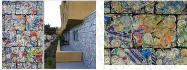
Gambar 2.35 Pengolahan kaleng bekas berupa blok-blok bata Brooks and Scarpa Architects Broadway Housing, Santa Monica, CA Sumber: http://inspirationgreen.com/aluminum-can-construction.html
