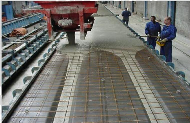
**Gambar 2.1** Pengecoran beton SCC
